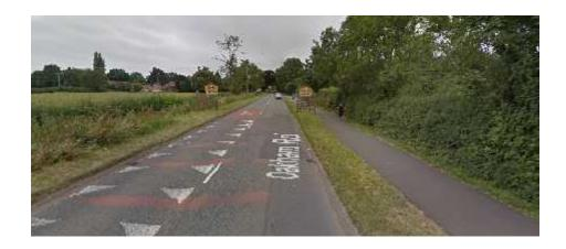
Throughout the village there are various traffic calming features, such as red friction surfacing with SLOW markings and speed indicator devices. The geometry of the road also lends itself to traffic calming through two tight bends. Examples of the traffic calming features in Langham are shown below:
