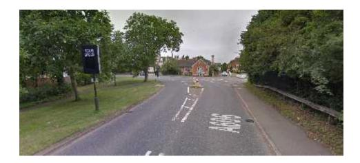
West of Burley Road junction, there is a solid white lines system, until just north of Cold Overton Road. There are no pedestrian crossing points along this section of road. There is a footpath on both the north and south side of the carriageway. The footpath on the south is 1.2m wide and the footpath on the north side is 1.8m wide, however is reduced at some locations due to overgrown vegetation.
